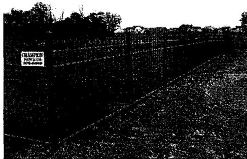
2.15.2 Dimensions: Fence pickets should be at least forty-two (42) inches and cannot be taller than seventy-two (72) inches. The picket height is measured from the ground to the tallest picket. The vertical posts should be slightly taller than the pickets. The fence should not have more than 70% of its surface closed. The spacing between the closed surfaces (pickets) must equal at least 30% of the picket width plus the space between.
